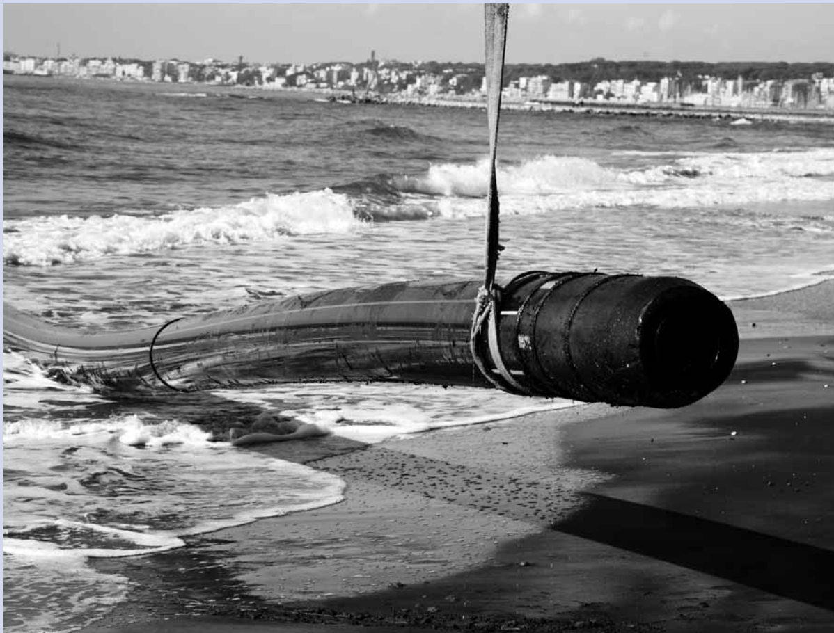
The SA.PE.I. cable at the Latina end.
