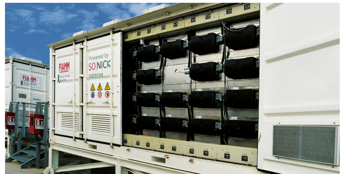
Storage Lab – Codrongianes: Battery container details – ZEBRA technology
